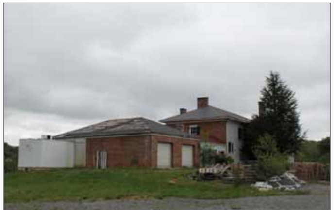
Current condition to the Denton House.
