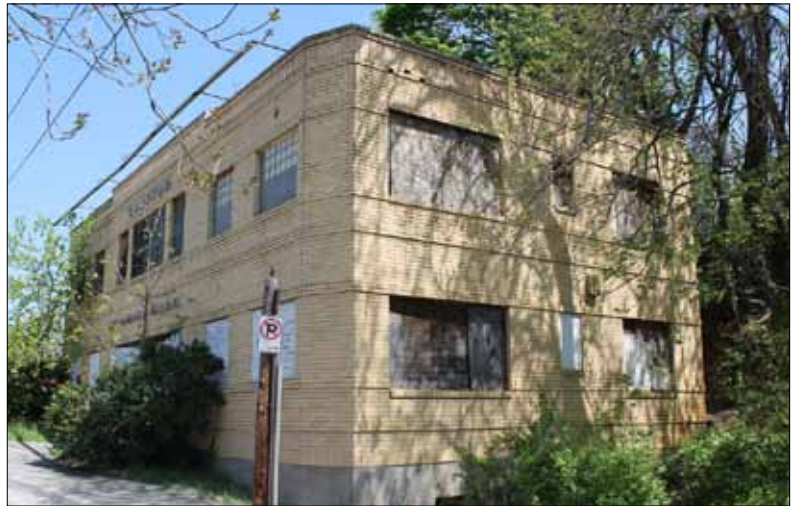
Current condition of Claytor Memorial Clinic.
