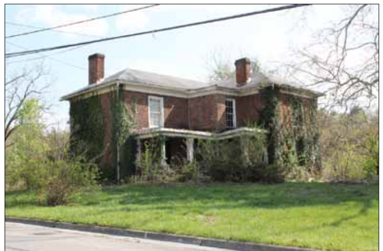
Riverdale prior to demolition of porches in April 2013.
