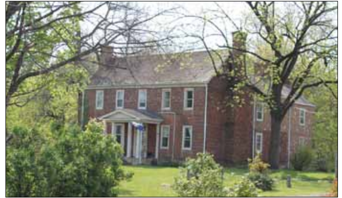
Current condition of the Preston House.
