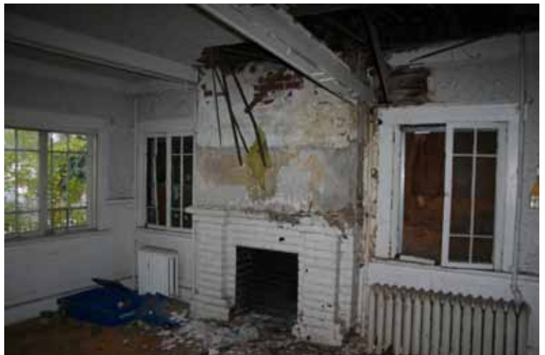
Interior prior to renovation.
