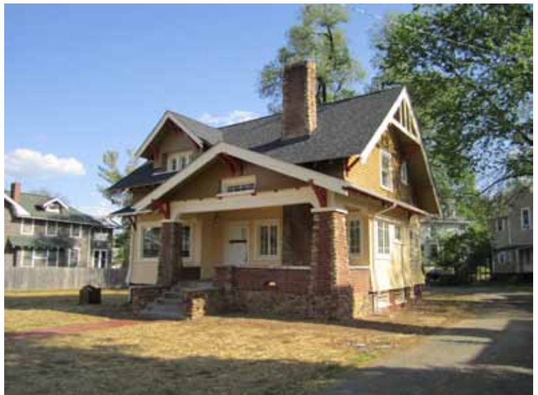
Front elevation post renovation. All photographs courtesy of John Garland
