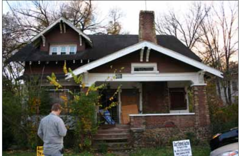
Front elevation prior to renovation.
