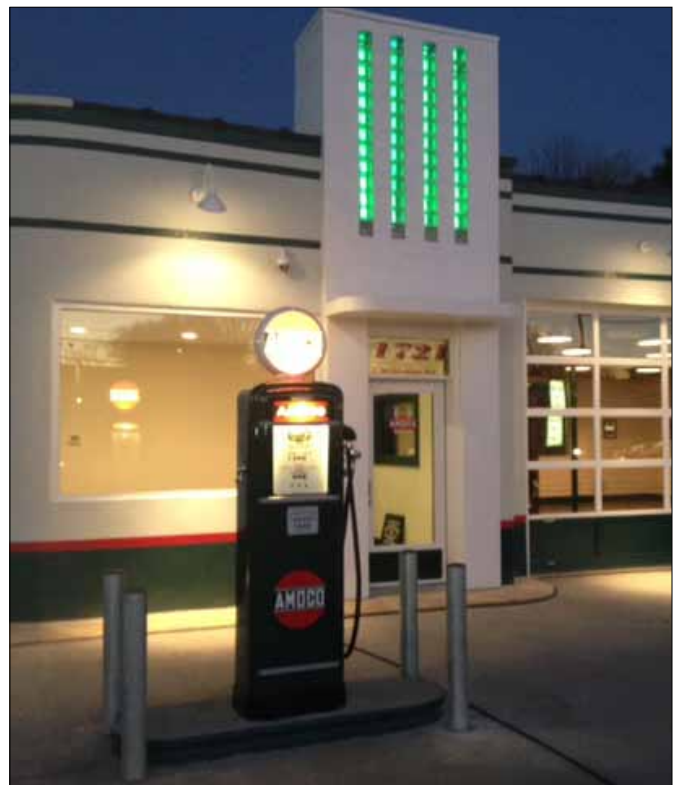
Entrance pylon with illuminated glass block. Photograph courtesy of Berglund Automotive Group
