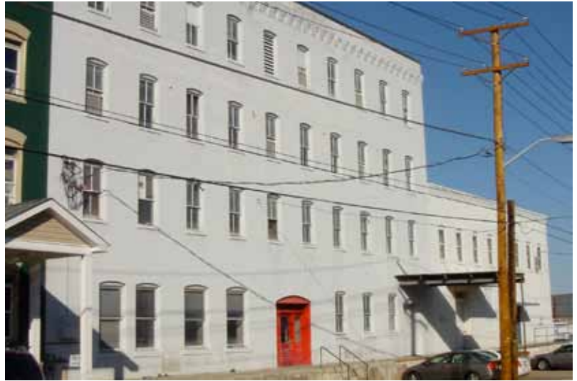
Front elevation prior to renovation.
