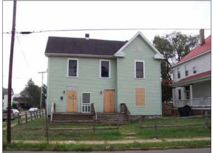
1602 Salem Ave. prior to renovation.
