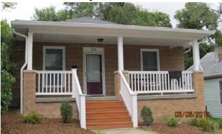
New construction at 29 14th Street.
